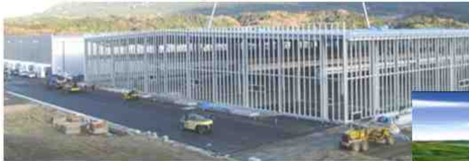
Progress of New Assembly Factory
